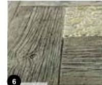
Stamped concrete - Woodgrain (Walkways over dry creek)
